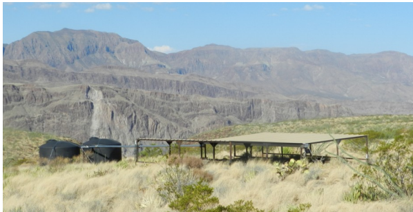
A typical guzzler consisting of a catchment, diversion pipe, water storage tanks, and trough.
