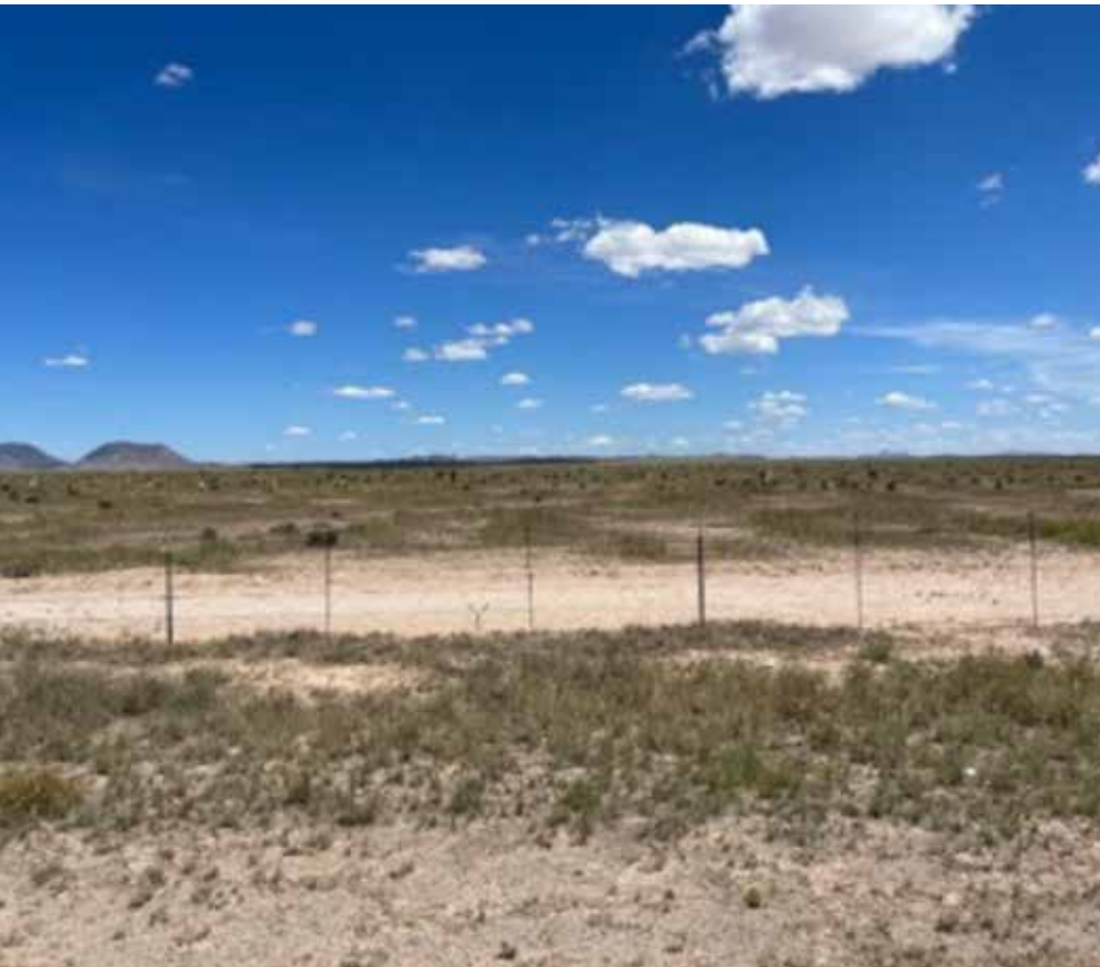
Figure 3: An example of a wide fence set-back along the roadway with pronghorn-friendly fencing. This situation would allow animals to more easily clear the roadway when vehicles approach. The bottom wire of the pronghorn-friendly fencing is 18-20 inches from the ground, allowing pronghorn to pass easily underneath.
