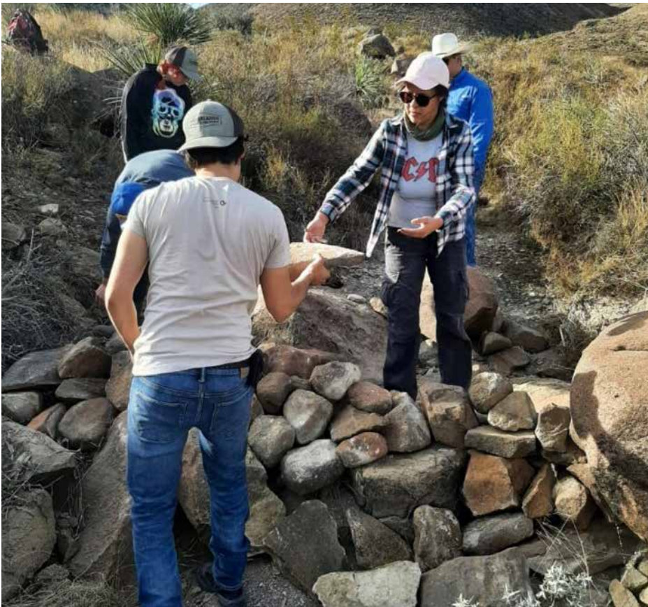
Undergrads from Sul Ross State University helped BRI researchers construct trincheras at a private property in Brewster County. Nearly 150 of these structures were set and assessed during 2022 and 2023.
