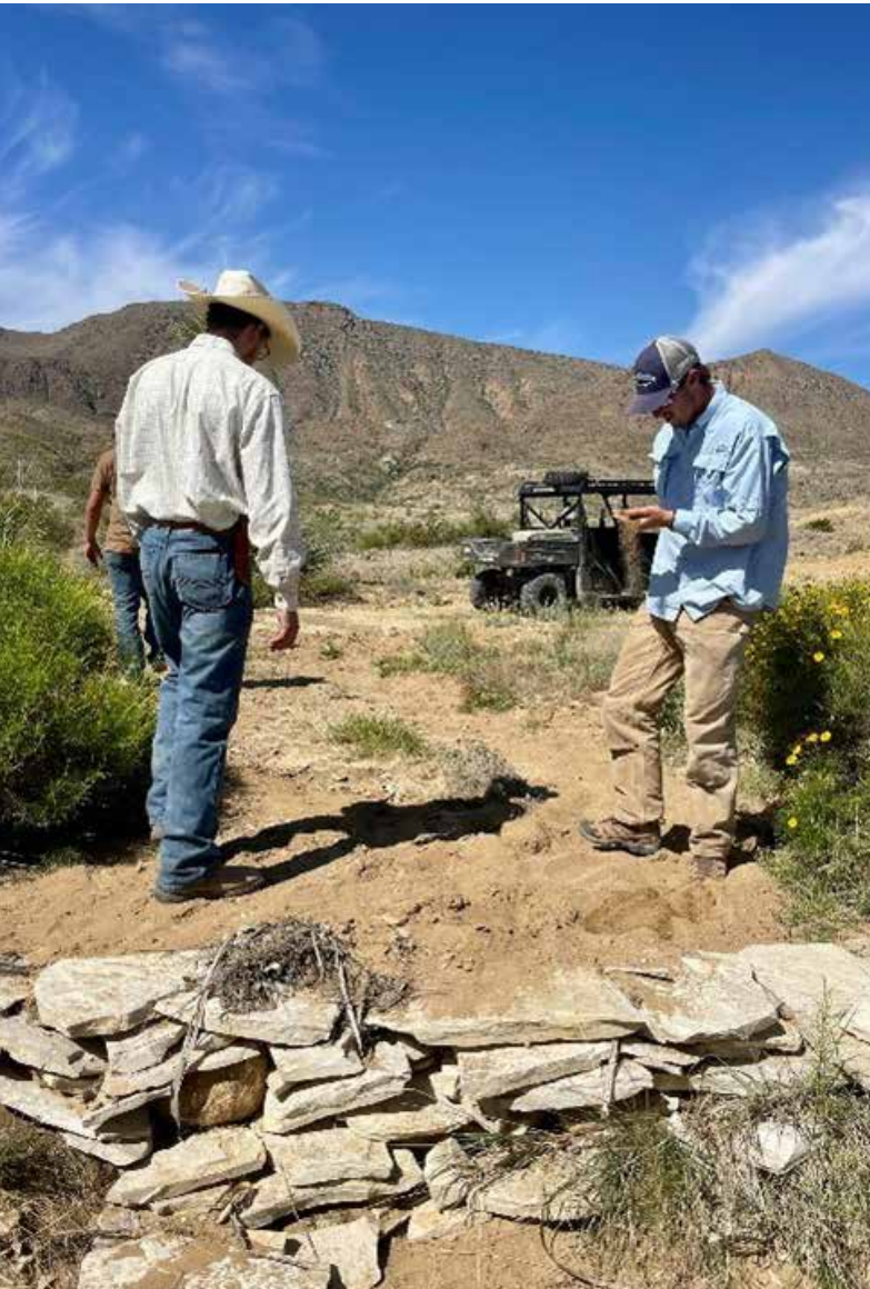
After two years, a significant amount of sediments were trapped by the trincheras. Monitoring will continue to assess plant cover changes and soil accumulation patterns.
