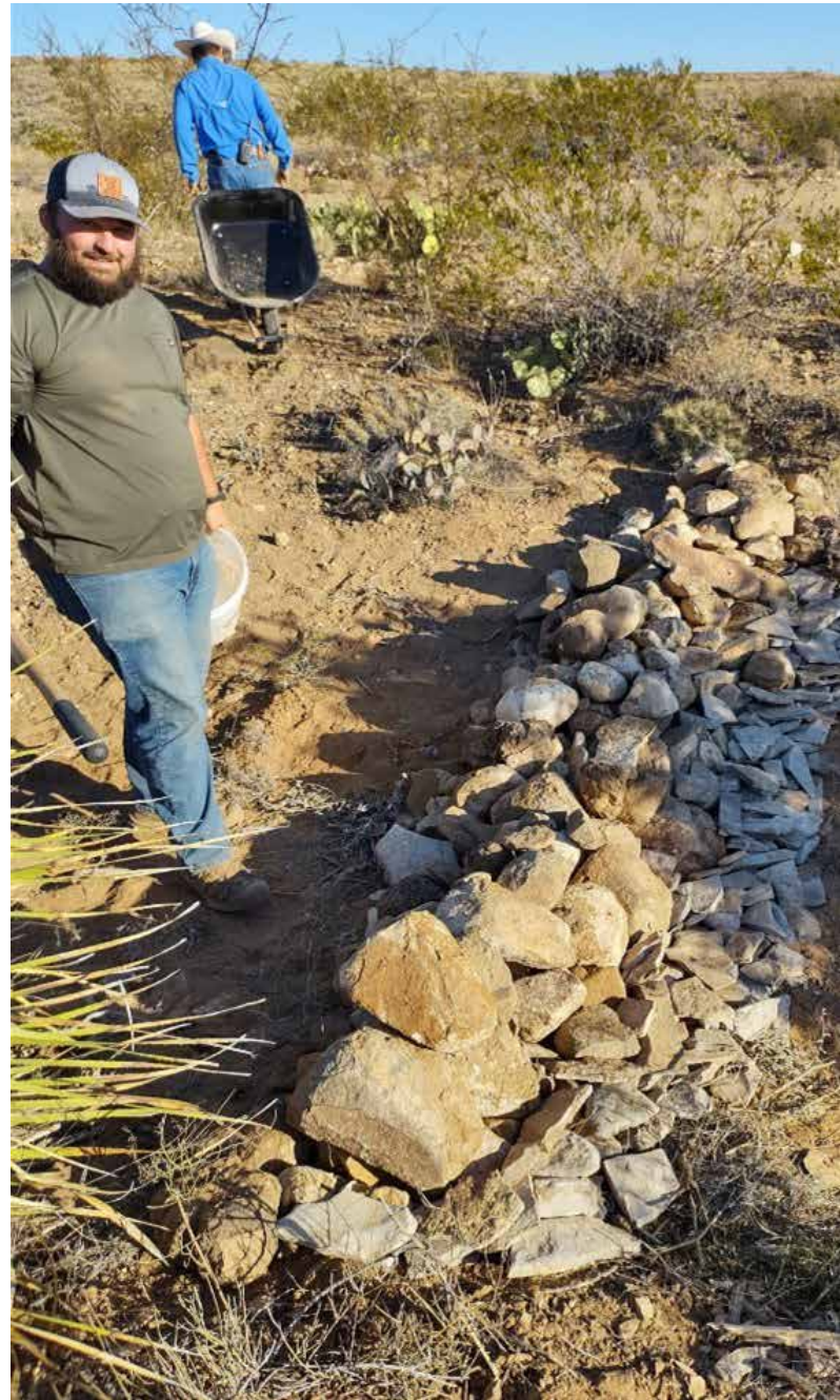
After two years, a significant amount of sediments were trapped by the trincheras. Monitoring will continue to assess plant cover changes and soil accumulation patterns.
