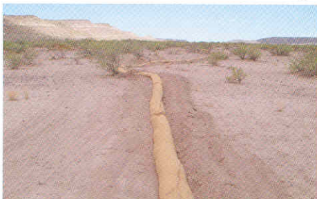
Dozed wattle treatment immediately after installation, July 2006, and one year later, August 2007.
