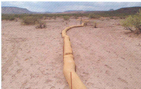
Staked wattle treatment immediately after installation, July 2006, and one year later, August 2007.
